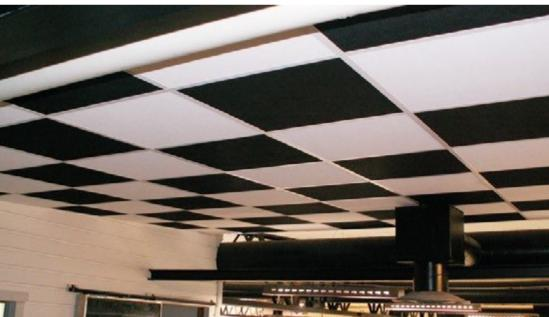
After installing the T-24 carrying system for ceiling panels, you may need simple 60x60cm Tiles for ceiling, it is common to use the gypsum board ceiling, but for those who are looking for higher acoustic solution and much more aesthetic improvement, the normal gypsum board will not be enough, therefore we offer Acoustic ceiling panels made of GlassWool coated anti flame paint available in any color.
