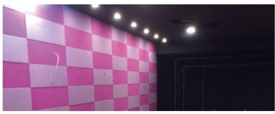
Acoustic panel made of rockwool and coated acoustic fabric, for installation we developed unseen screws system for easy installtion to the wall without necessarily need of a metal frame in the wall.
